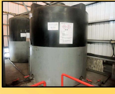
To prepare the coating, liquid chemicals are stored in large vats ready to be filled with crushed salts.
